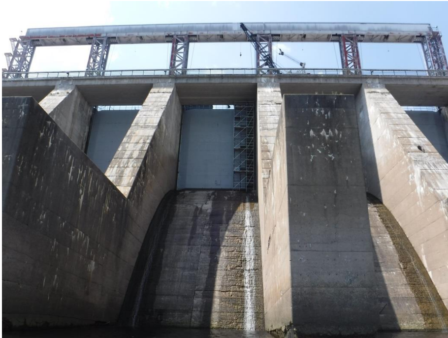
Above: Spillway gate under repair.
