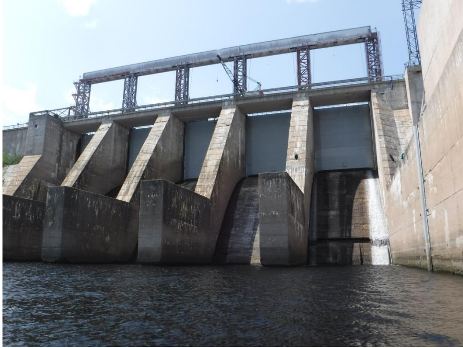
Above: Main Spillway with all gates closed.
